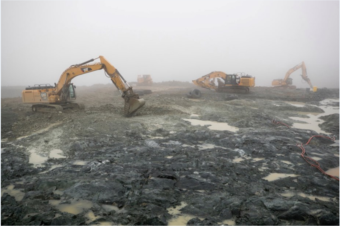
Preparation of the foundation rock, Photo Credit: Ken James, DWR
