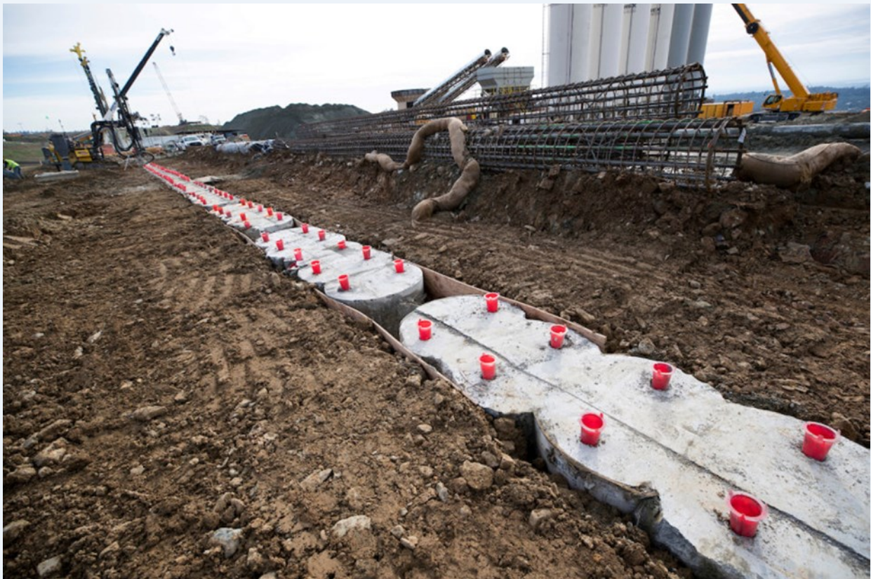
Secant Pile or Cutoff Wall, Photo Credit: Ken James, DWR
