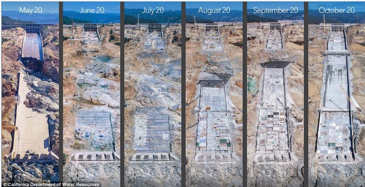
Repair Progression, Photo Credit: DWR
